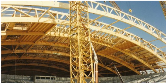
Figure 2. Construction of Atlantic Pavilion May 1997 (Courtesy of Instituto Superior Técnico).
