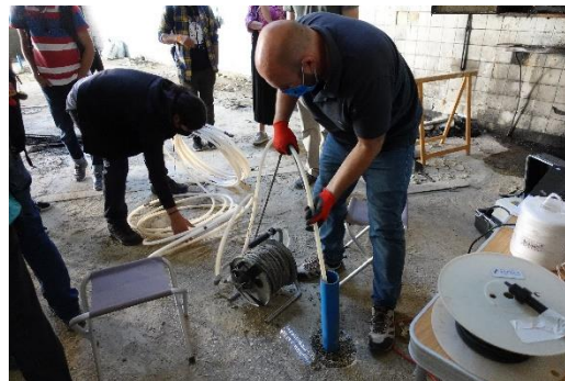
Figure 2. Pumping test in Lisbon downtown during COVID pandemic.
