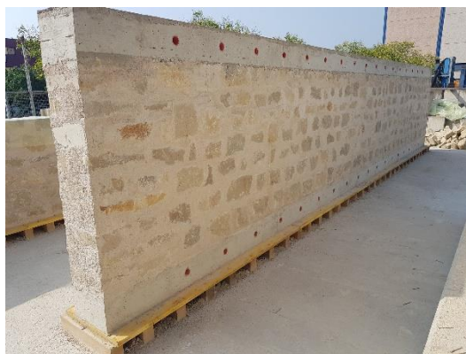
Figure 1. Unreinforced (bare) slender pier and wallets for characterization under vertical compression.
