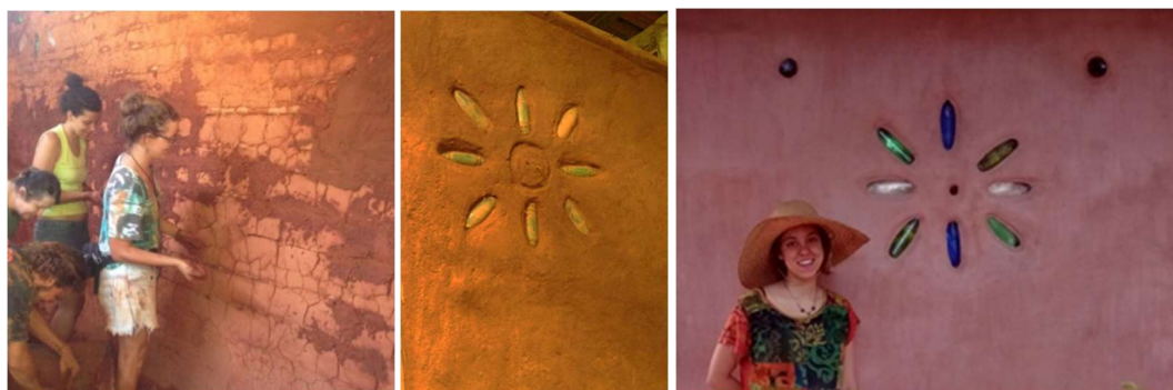
The cow dung addition on clay plasters reduces shrinkage, improve water resistance and provides a better finishing for renders.
