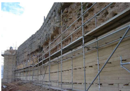
New rammed earth in heritage conservation site.
