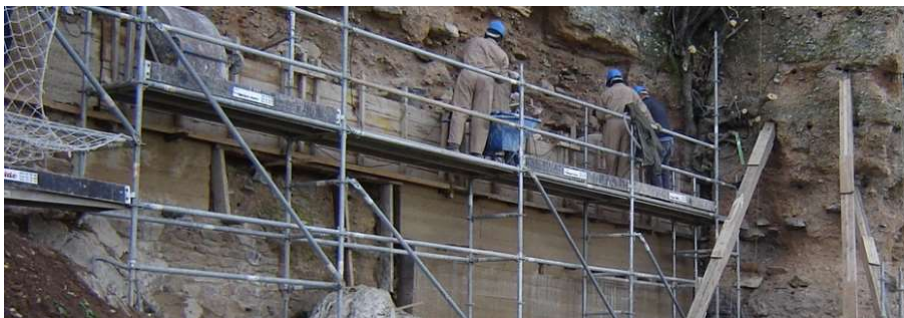
Heritage rammed earth repair and conservation.
