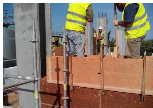
New rammed earth in a new construction site.
