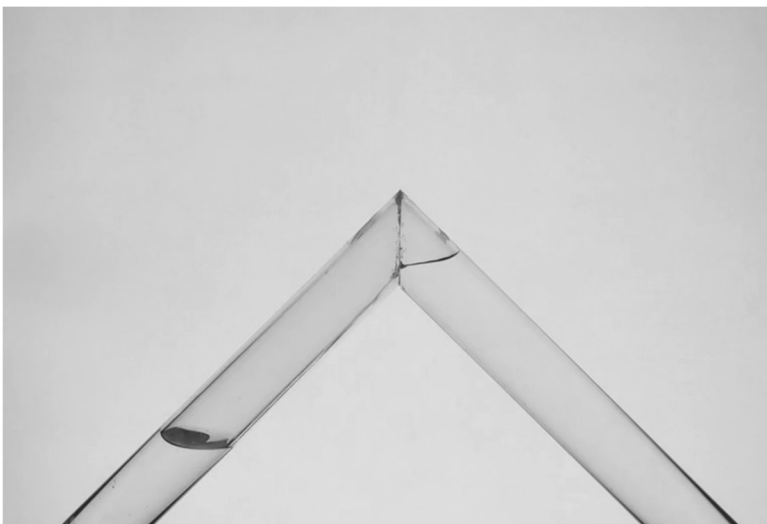
Entrapped air pocket in pipe.
