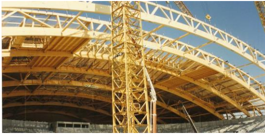
Figure 2. Construction of Atlantic Pavilion May 1997 (Courtesy of Instituto Superior Técnico).
