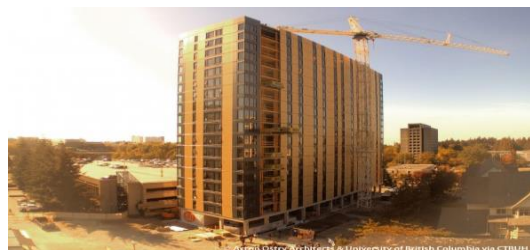
Figure 1. ‘Brocks Commons’ Vancouver, Canada. 18 Story Building (Acton Ostry Architects Inc. & University of British Columbia).
