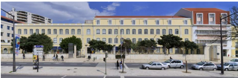
Figure 1. Building A, Lusófona University– Lisbon University Center.
