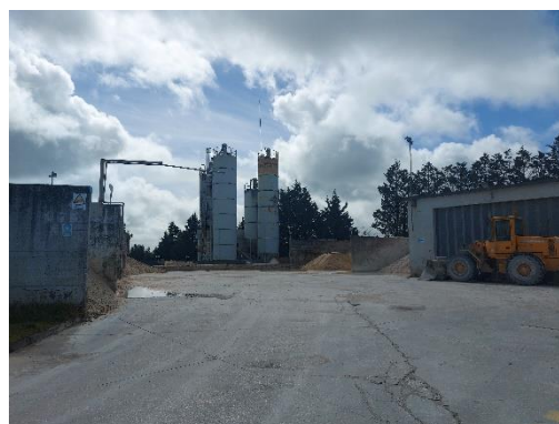
Figure 3. Ready mixed concrete plant.
