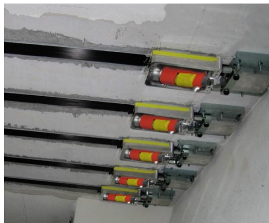
Figure 1. CFRP laminates for strengthening RC structures.
