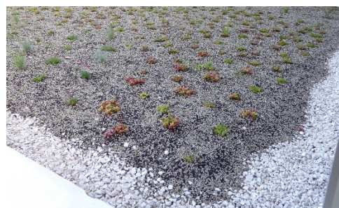
Figure 1. Functional prototype of a green roof installed in the Itecons building in Coimbra.
