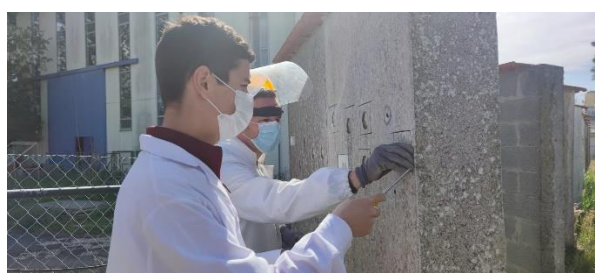
Figure 2. Pilot applications of ETICS and protective solutions at walls prototypes.
