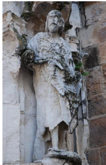
Figure 1. Example of a degraded statue in a porous carbonate stone.
