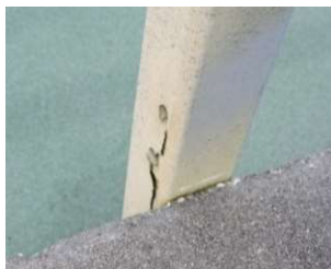
Cracking
