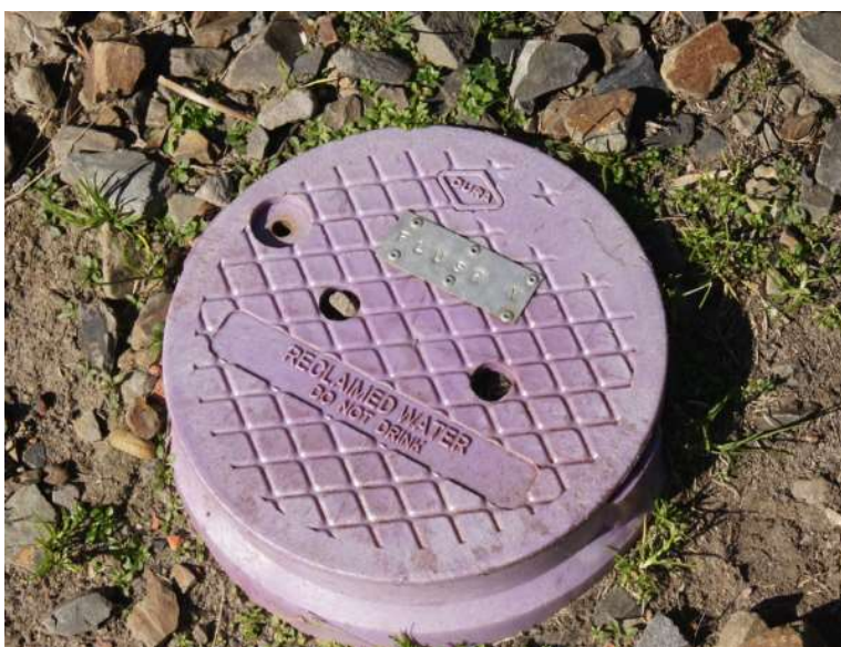
Reclaimed water – an alternative water resource identified by purple color.
