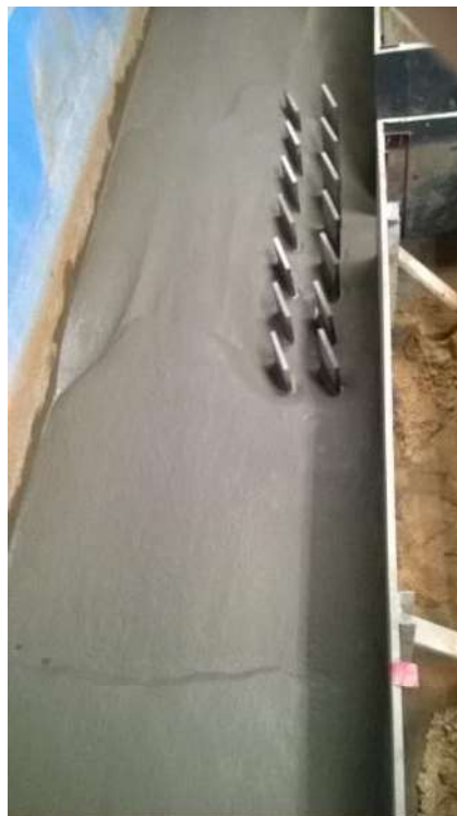
Vane-field in front of the diversion channel.
