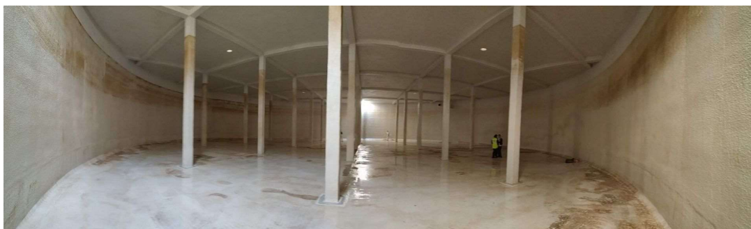
Interior view of a circular cross-section water storage tank.
