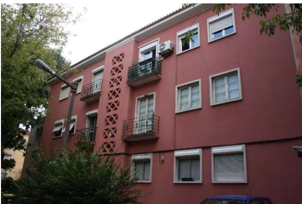
Type of mixed masonry-reinforced concrete "Placa" buildings.
