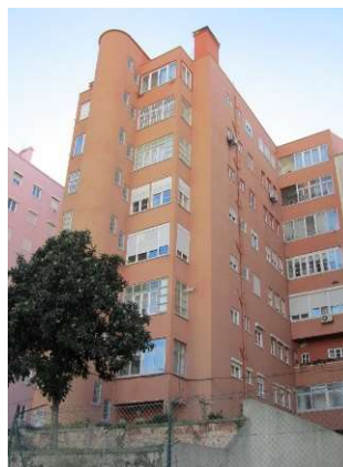
Type of mixed masonry-reinforced concrete "Placa" buildings.
