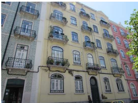
Unreinforced masonry buildings constructed in the beginning of the 20 th century in Lisbon.
