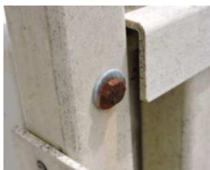
Corrosion of bolted elements
