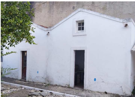
Building envelope inspection.
