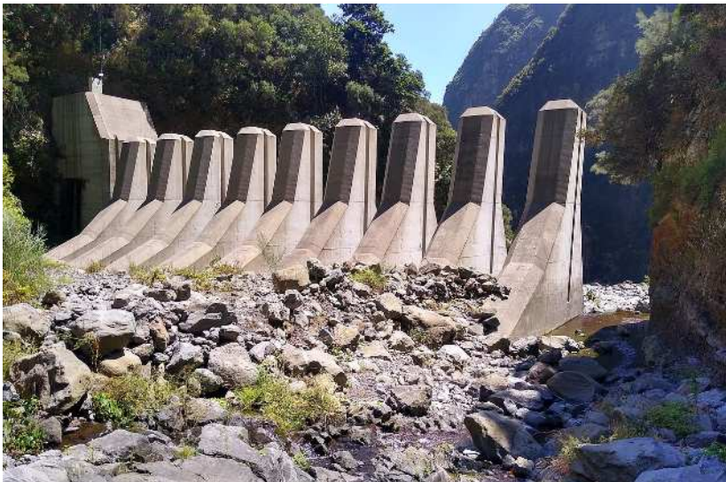
Open type check dam: concrete slit barrier of St. Luzia River in Madeira, Portugal.
