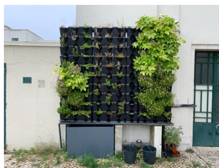
Figure 1. Urban Lisbon Living Lab logo and green wall for grey water treatment installed at IST.
