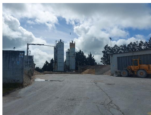
Figure 3. Ready mixed concrete plant.
