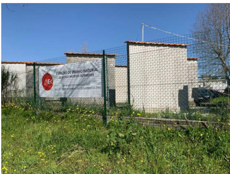
Real application of three render mortars with industrial wastes incorporation.
